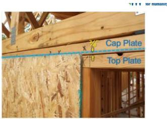
Figure 6-2. Wall Sheathing Set 1/2-inch Above Top Plate
